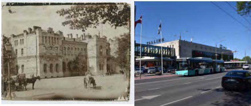
Figure 4: Baltic Station in 1900 (left) and 2024 (right)
